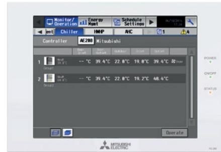
Centralized controller AE-200E
